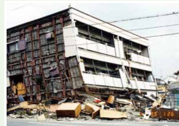
Collapsed Apartment Building (Great Hanshin Earthquake, January, 1995)
